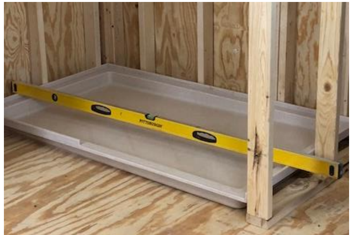
Level on top of water dam (Step 9)
