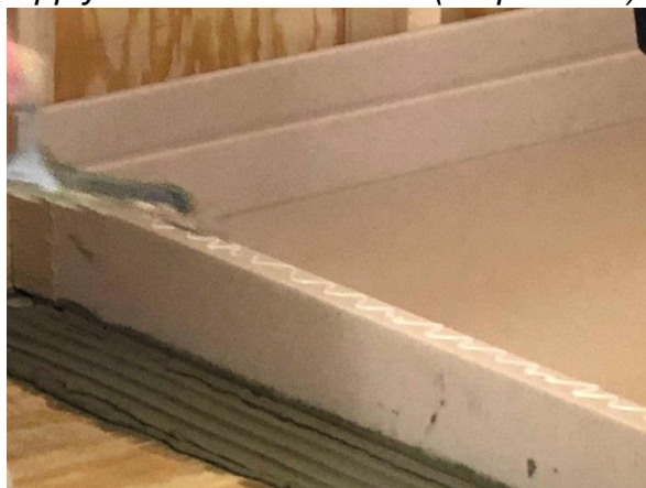
Apply Thinset and Sealant (Steps 5 & 7)
