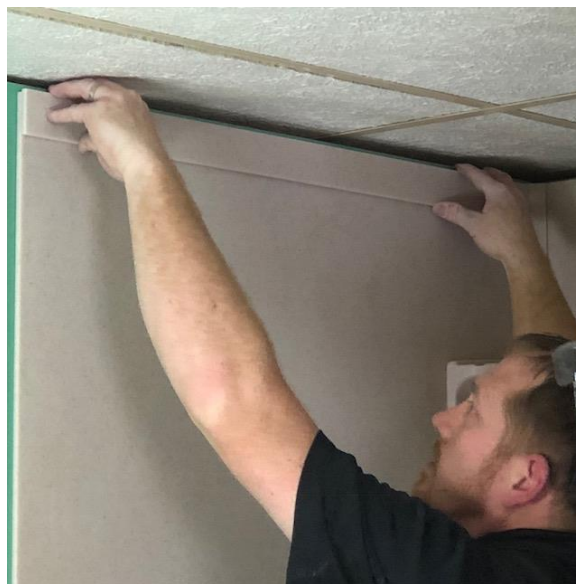
Install Batten at top of panel. (Step 5)
