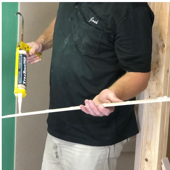
Apply adhesive to trim molding (Step 4)
