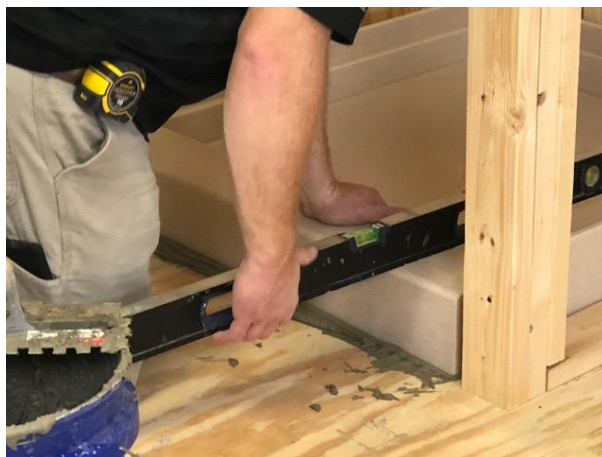
Level on top of Threshold (Step 9)
