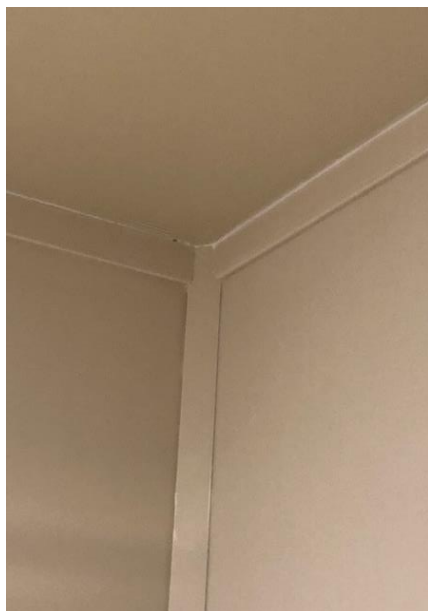
Batten at Inside Corner Mold
