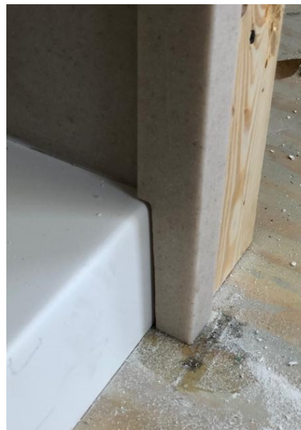
Outside Corner Mold at Base
