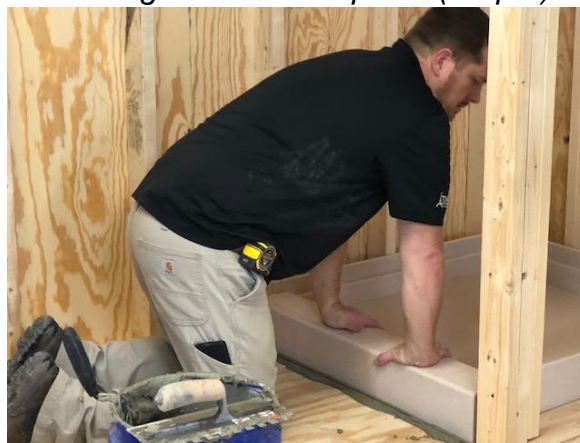
Setting Threshold in place (Step 8)
