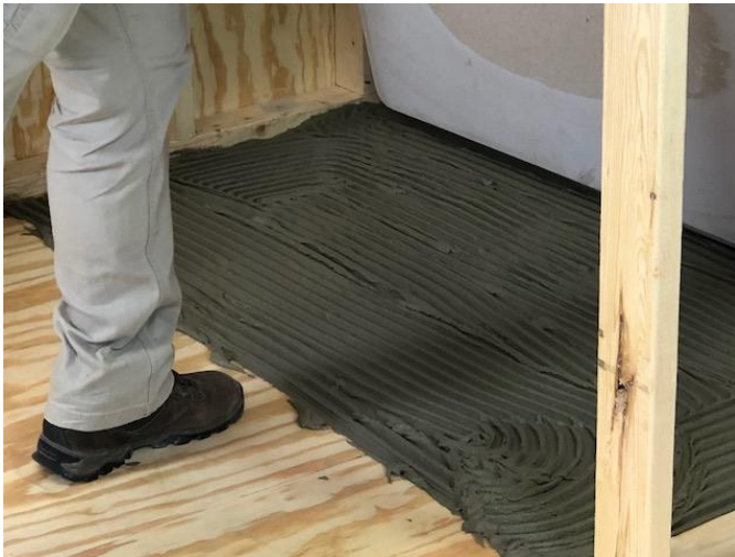
Apply Adhesive using 1/2" Notched Trowel (Step 8)
