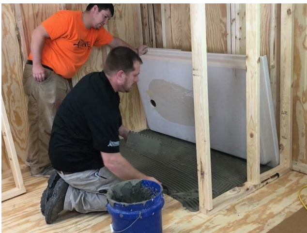
Shower Base being set in adhesive (Step 9)
