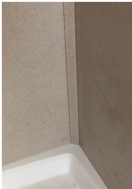
Inside Corner Mold at Base
