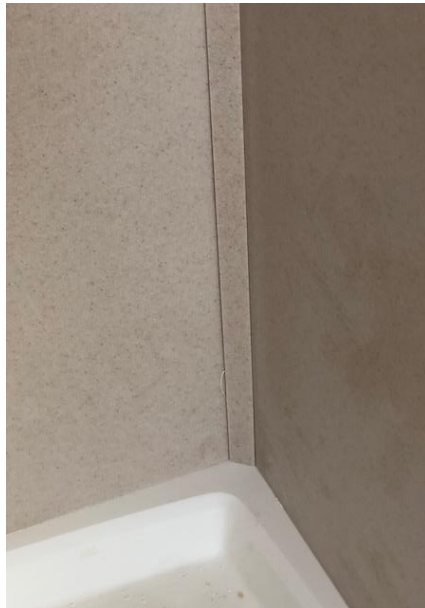
Inside Corner Mold at Base
