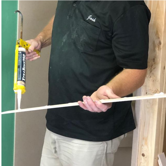
Apply adhesive to trim molding (Step 4)
