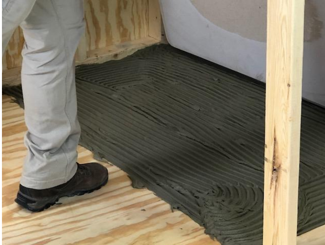
Apply Adhesive using 1/2" Notched Trowel (Step 8)
