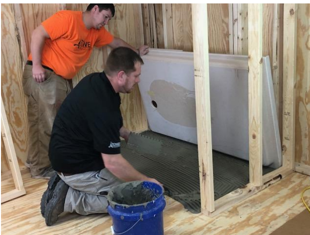
Shower Base being set in adhesive (Step 9)
