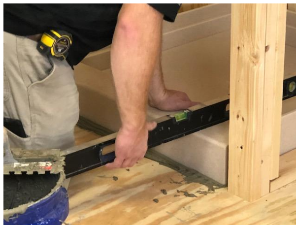
Level on top of Threshold (Step 9)
