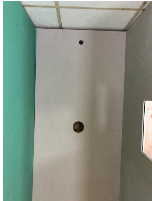
Holes for Shower Fixtures
