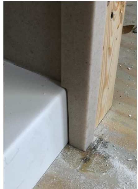
Outside Corner Mold at Base
