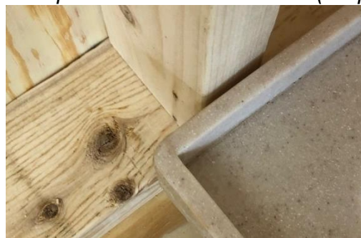
1/8" Gap between wall and base (Step 4)
