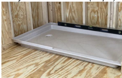
Dry Fit Base and Level (Step 4)
