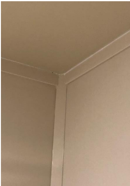
Batten at Inside Corner Mold
