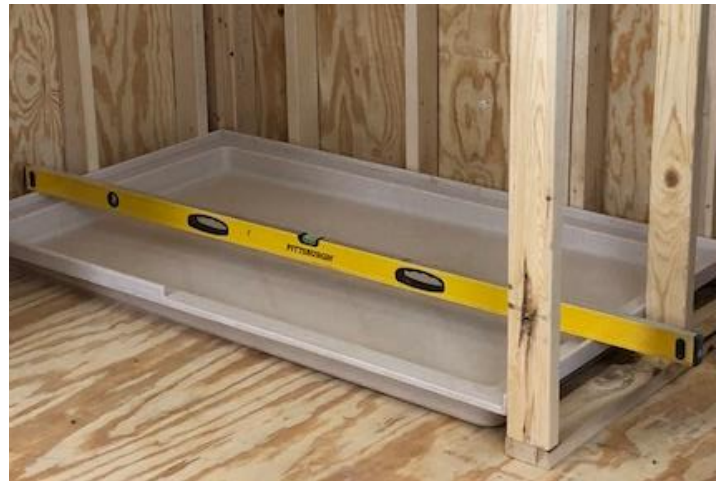
Level on top of water dam (Step 9)
