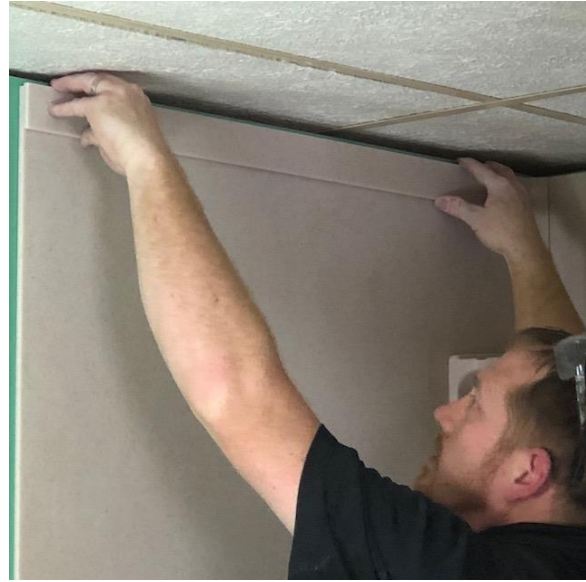
Install Batten at top of panel. (Step 5)
