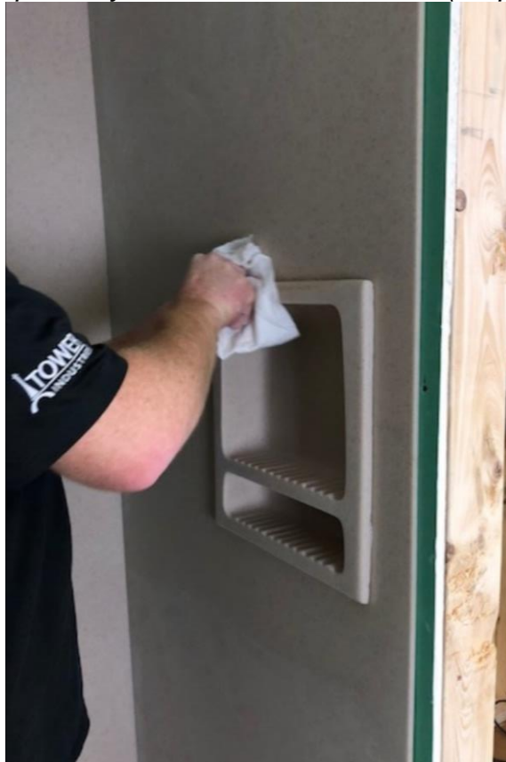
Wipe Away Adhesive around Holder (Step 6)
