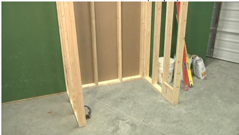
Clear area of all debris (Step 2)
