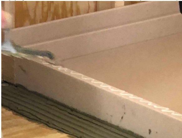
Apply Thinset and Sealant (Steps 5 & 7)
