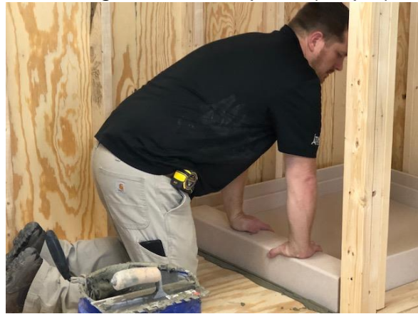
Setting Threshold in place (Step 8)
